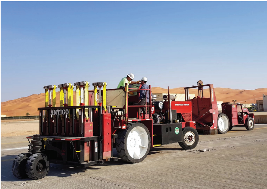
Figure 3: Multihead breaker and hammer guillotine in action at Shaybah Airport Runway.
