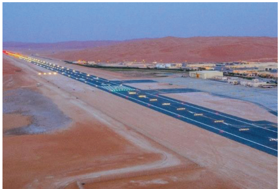
Figure 2: New Shaybah Airport Runway pavement after implementation of rubblization and overlay with polymer modified hot mixed asphalt (HMA).
