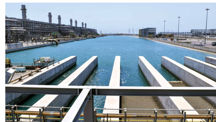
Oil refineries convert oil's hidden mysteries into finished hydrocarbon products, and the constant flow of the Red Sea through inlet and outlet channels at Jazan reminds workers of the importance of protecting the natural environment from harm.
