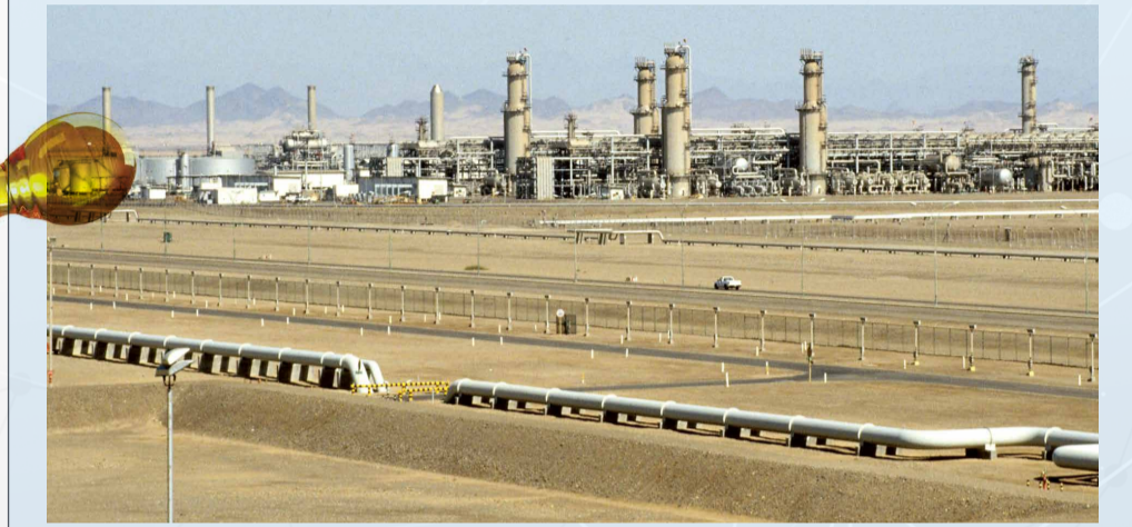
Routine flaring is significantly reduced at Yanbu' by diverting recovered ethane to be used as a fuel gas in boilers.
