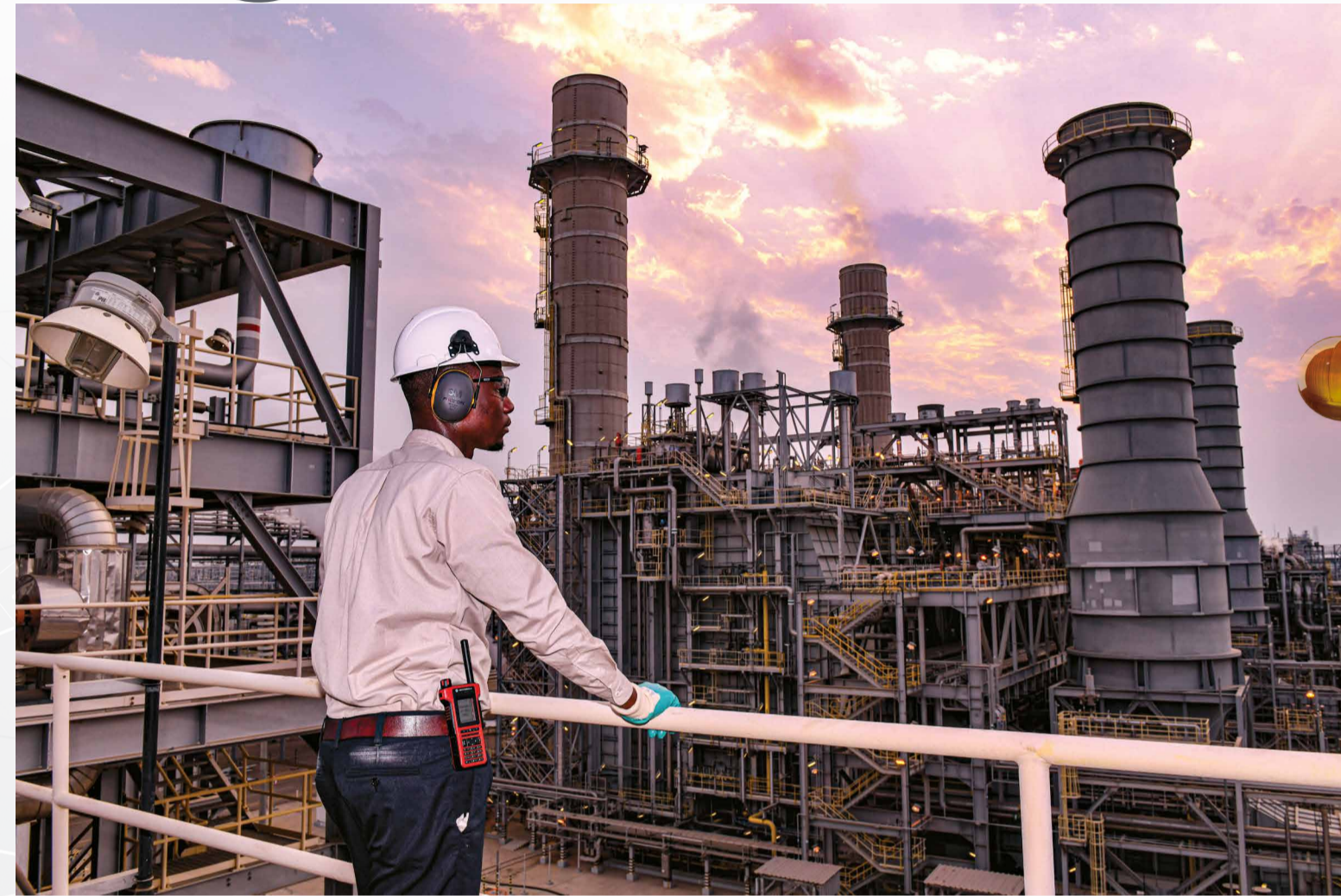
From an offshore mooring, the Jazan Refinery Complex receives stabilized Arabian Medium crude oil from the northern oil fields.
